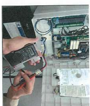
Fire Alarm Control Panel Checking Battery Voltage 24 Vdc
