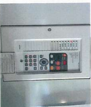
Fire Alarm Control Panel Testing.
