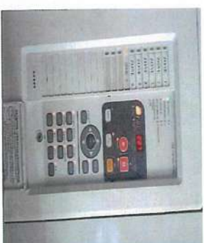
Fire Alarm Control Panel Testing.
